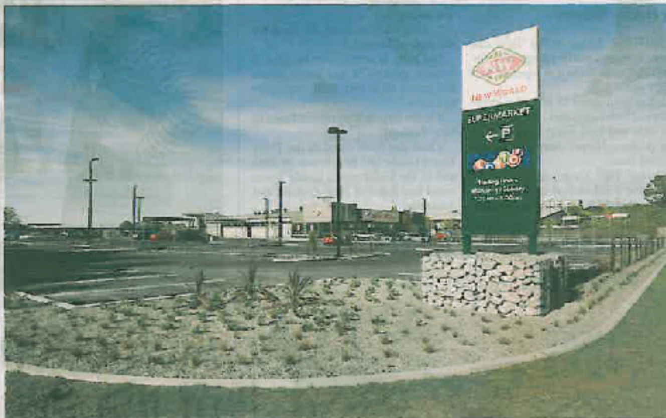
This New World supermarket is part of an urban development at Lincoln which aims to set high standards for sustainable land use.
